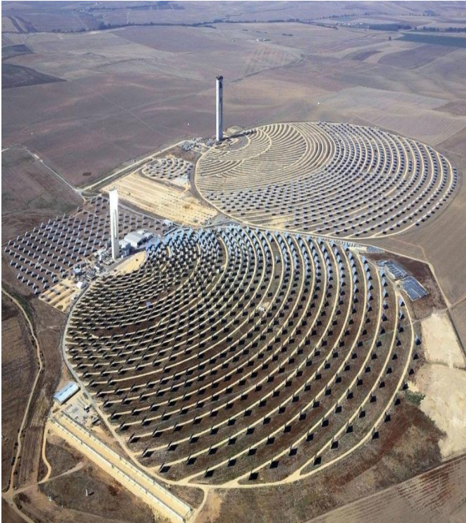
Figure 6: About twenty kilometers from the city Ouarzazate, the largest solar plant in the world is implanted.
